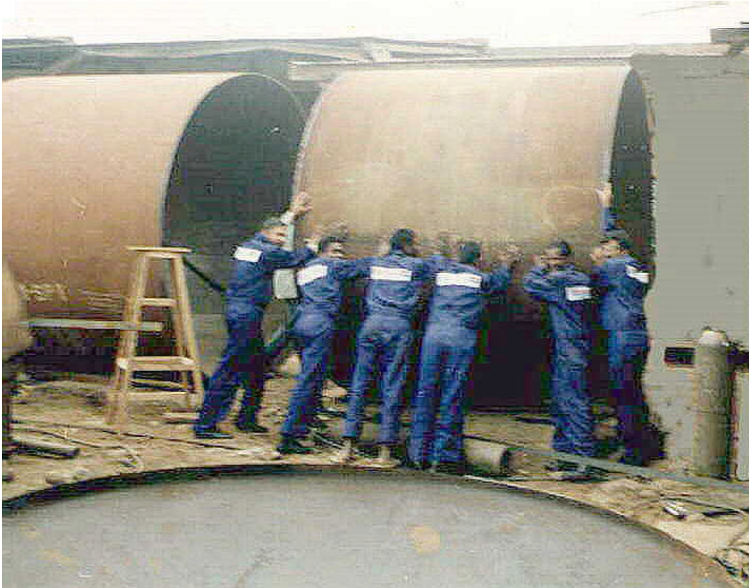
Bulk Oil Storage Tank Site Fabrication at Revoline Lubricants Kampala. Uganda.
