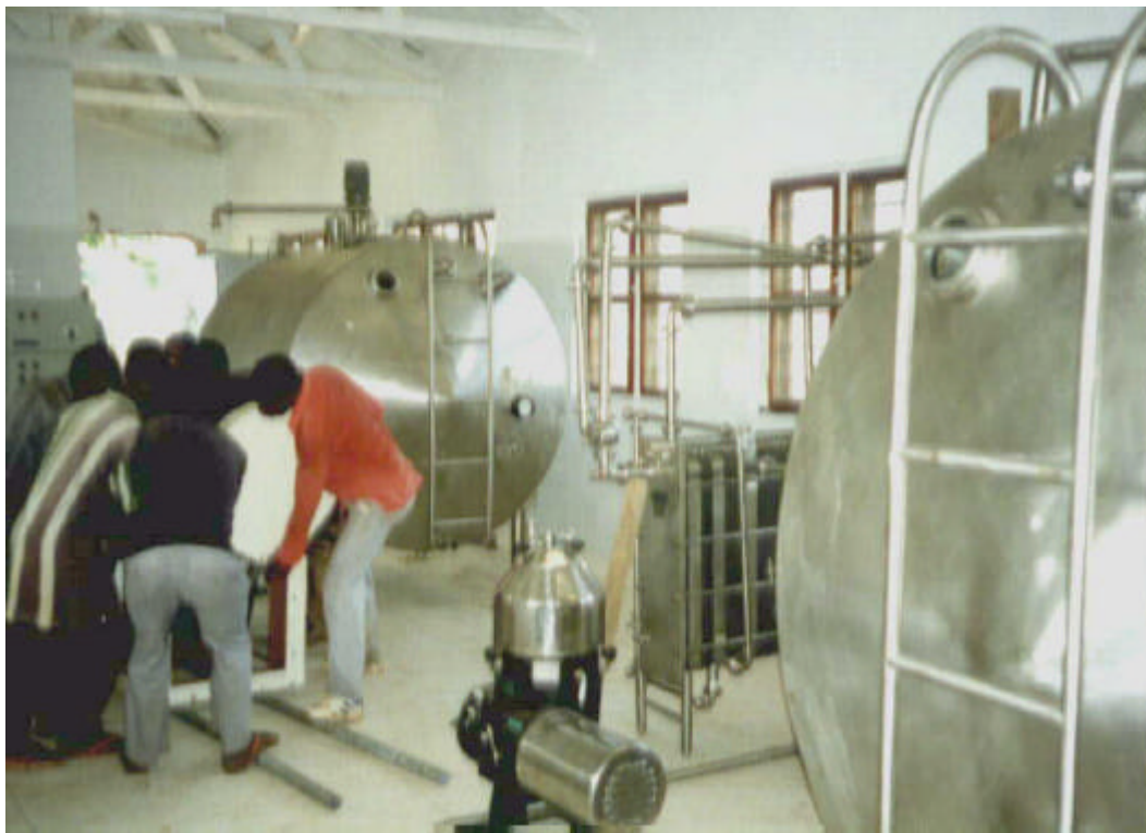
Sugar Mill Fabricated Tank under shipment from works. SS Fabricated tank for dairy plant under Installation in Tanzania.
