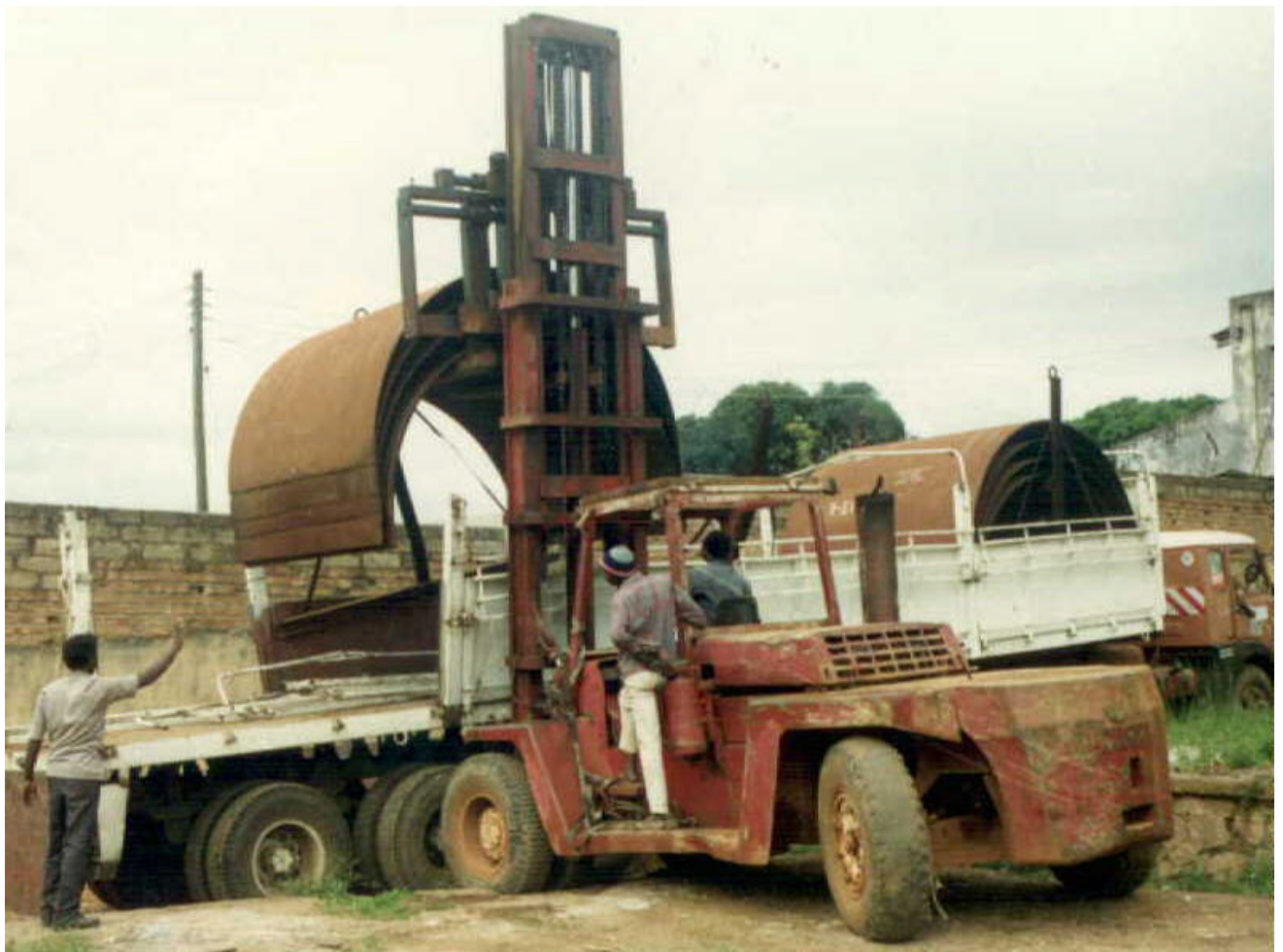
Tank Fabrication from CKD rolled plates
