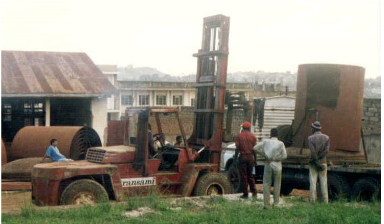
Tank Fabrication from CKD rolled plates.
