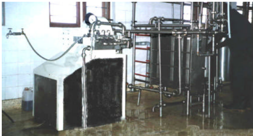
Homogeniser and Plate Pack pasteuriser
